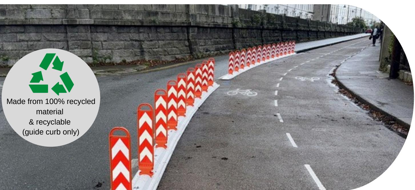
More than 100m of the truly mobile and flexible system was set down in Dun Laoghaire. The unique ARS anti-slip system sticks like glue to the road with no need for any typically damaging installation methods.
